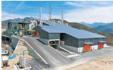
RKN Combines a pusher-type stoker with a countercurrent rotary kiln, for stable processing of waste with many different calorific values.
