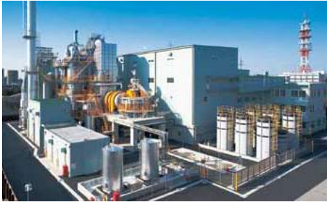
ISR Combines a stoker incinerator and a rotary kiln incinerator. The water-cooled walls let it recover heat and generate power.
